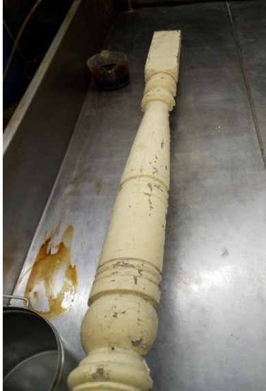
Figure 2: Decorative column with lead-based paint
